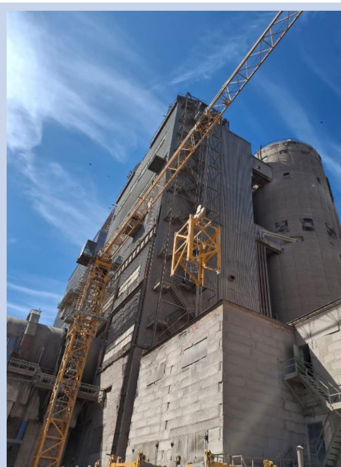
New crane for Line 6 preheater tower.
